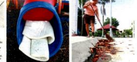
At Jalan 17/15, playground equipment is in a state of disrepair and is a danger to children and adults alike. - AFP/ The Star
